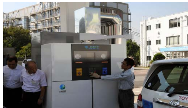
Start refueling of 70 MPa hydrogen
